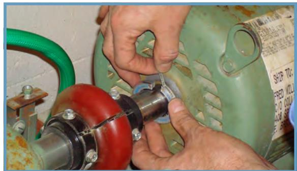
Next, the ring was pushed back against the bare metal of the end bracket, maximizing electrical contact via the conductive epoxy. To ensure that the ring was correctly centered around the shaft, small metal spacers (included in the kit) were inserted into the gaps between the two halves of the ring. Once the adhesive cured, the spacers were removed. The entire installation took about 10 minutes.
