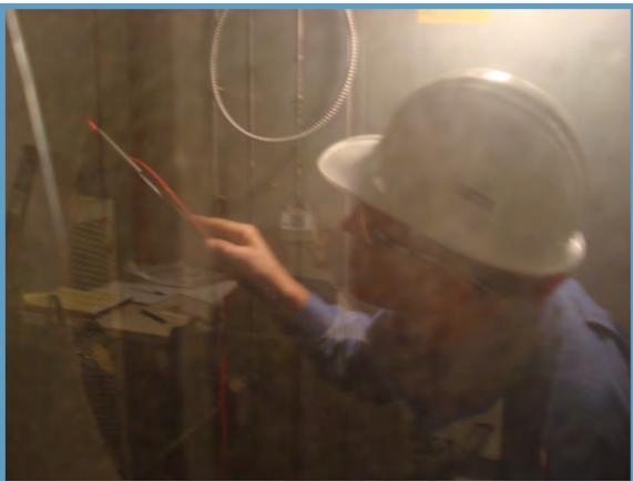
The shaft was cleaned and prepared in the same manner as that used for Motor #1, but because the motor shaft was difficult to reach and only a couple of inches of it between the end bell and a sheave were exposed, the versatility of the split-ring AEGIS® SGR and the ease of installation using conductive epoxy became even more apparent.
